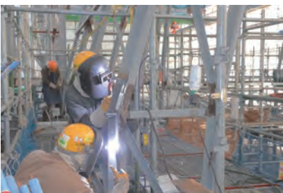
鉄骨溶接補修 (H29.11)
